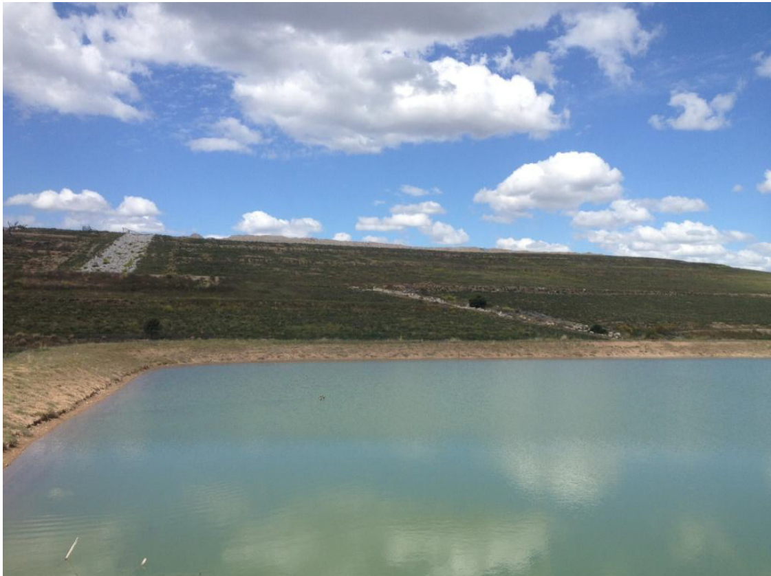
Figure 3 - Rock lined waterway on the southern emplacement
